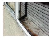
Evidence of problems resulting from condensation can be seen on the interior window sill.
