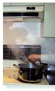
Use your kitchen exhaust fan or range hood to remove humidity generated by cooking. The exhaust fan should be vented to the outside.
