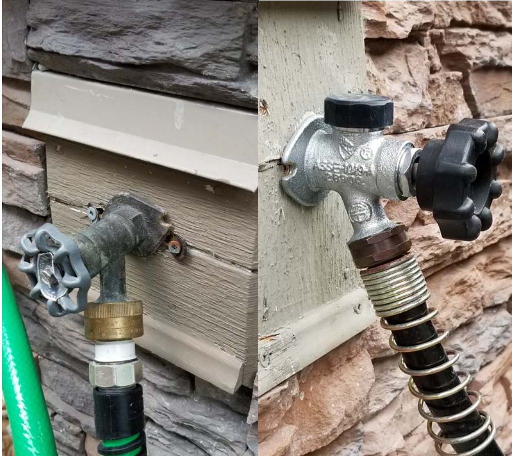
Examples of typical frost free design faucets. Identified by longer, larger, more robust body construction.
